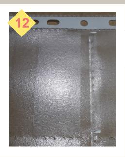
Set the flap min. 3mm above the weld. On the flap, make a weld on the existing weld on the envelope.
